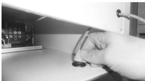
5. Seal the porthole with putty - both inside and outside.
